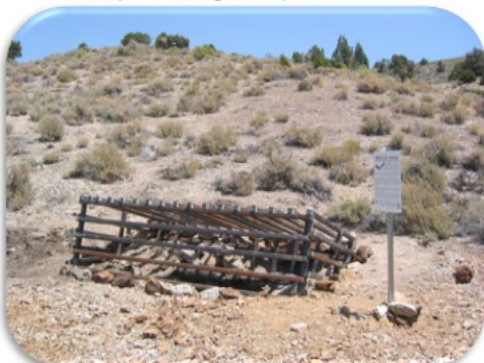
Bat compatible shaft copula - Unknown photographer
