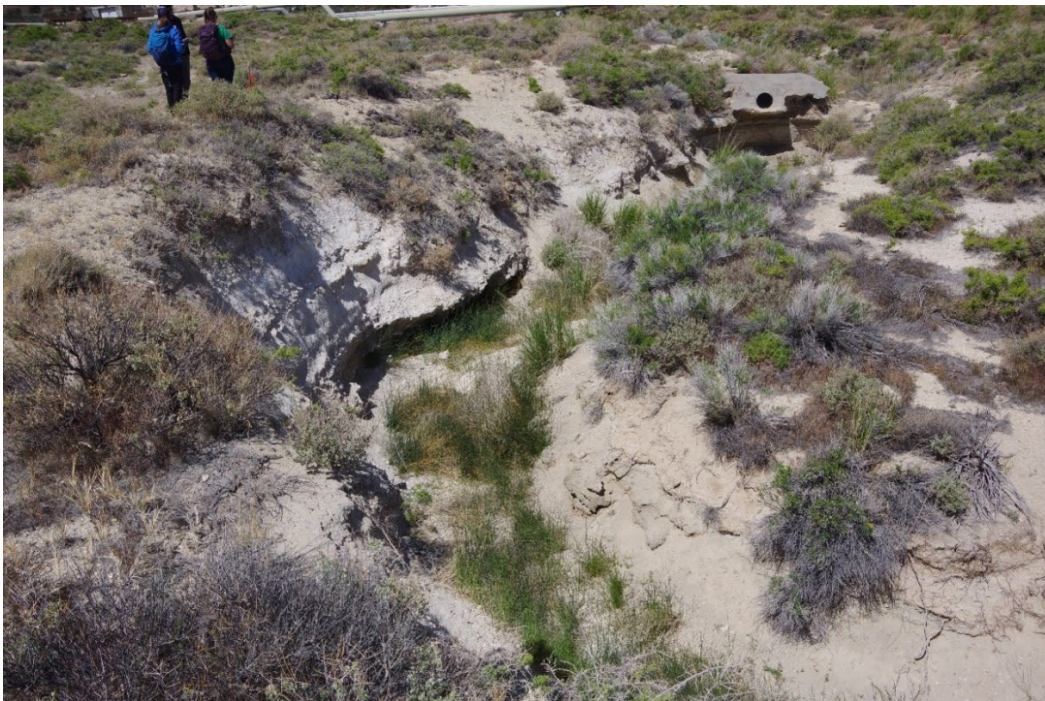
Photo 2a: Stream channel created by culvert near ORMAT operations. J. Johnson, NDNH botanist, May 13, 2022.
